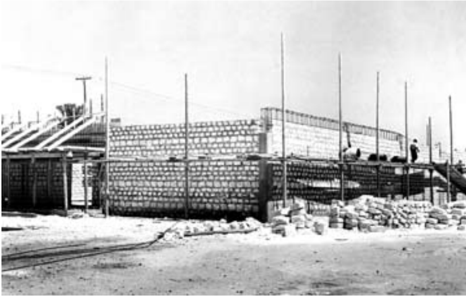
For the communications center, under construction at Wheelus Air Base in August 1951, native limestone blocks were placed to the first bond beam level and reinforced steel was used for a section of the bond beam.
