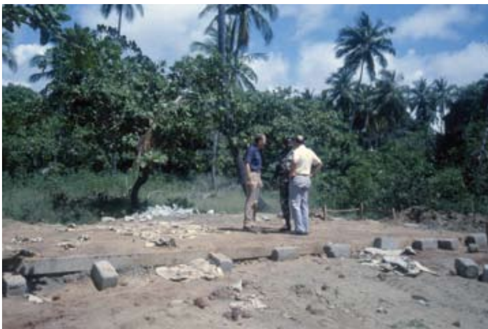
Project site in Kenya, November 1989
