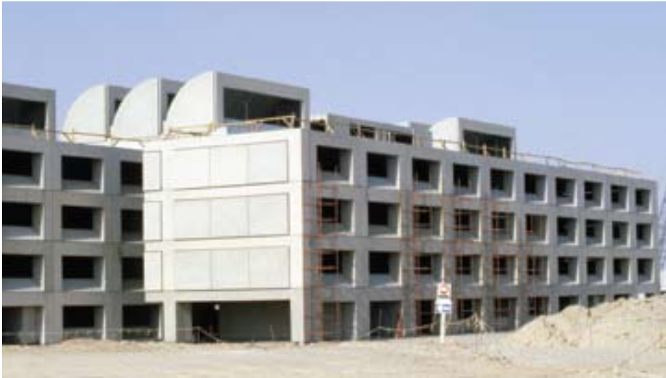
New bachelor enlisted quarters at King Khalid Military City, August 1981
