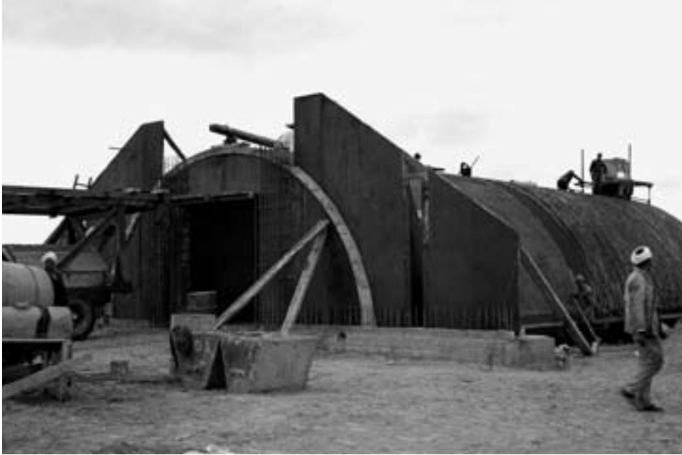
Construction of a storage igloo for ordnance at the Sidi Slimane air base, shown here in February 1957, was completed later that year.
