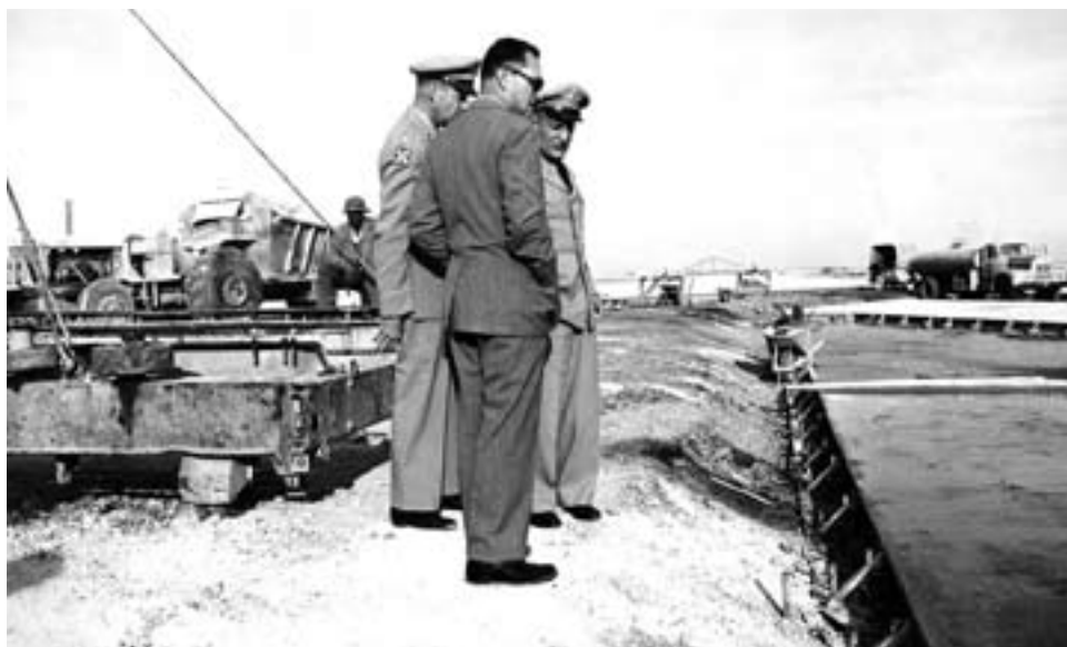
In September 1956, Chief of Engineers Maj. Gen. Emerson C. Itschner ( right ) visited Mediterranean Division headquarters at Nouasser, where he observed concrete paving of the taxiway with Lt. Col. John W. Chesley Jr., area engineer, and Paul Erskine of Atlas Constructors.
