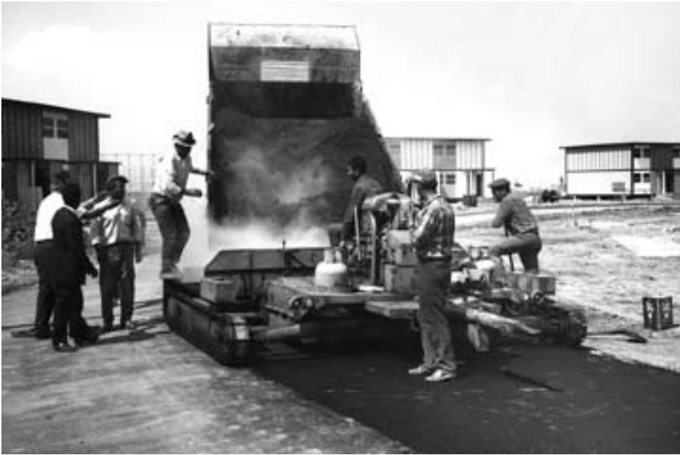
Asphalt paving during road construction in the family housing area at Karamursel, June 1970
