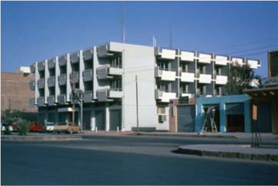
Saudi Arabia District Office, Riyadh, 1969
