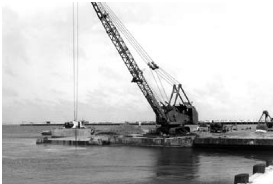
Chisimayu Port construction using a clamshell on a crane barge to remove underwater high spots, September 1966
