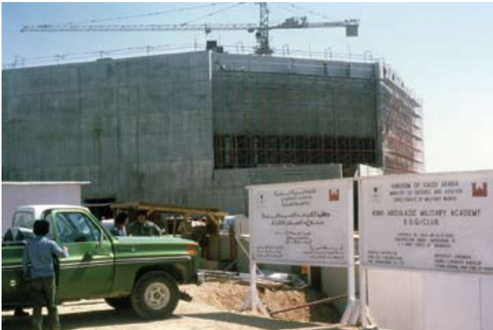
Construction of bachelor officers quarters and club at King Abdulaziz Military Academy, April 1982
