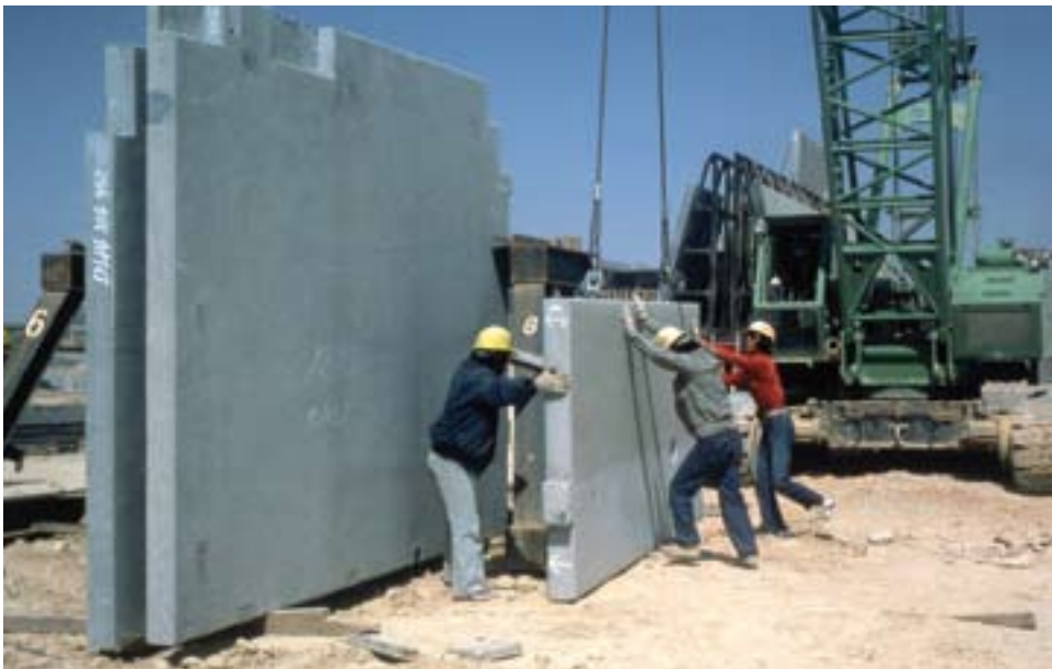
This page and top right, precast concrete panels were used extensively in construction at King Abdulaziz Military Academy.
