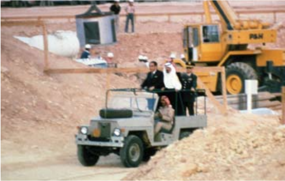
Prince Abdullah touring the construction site of the Saudi Arabian National Guard headquarters complex, 1977
