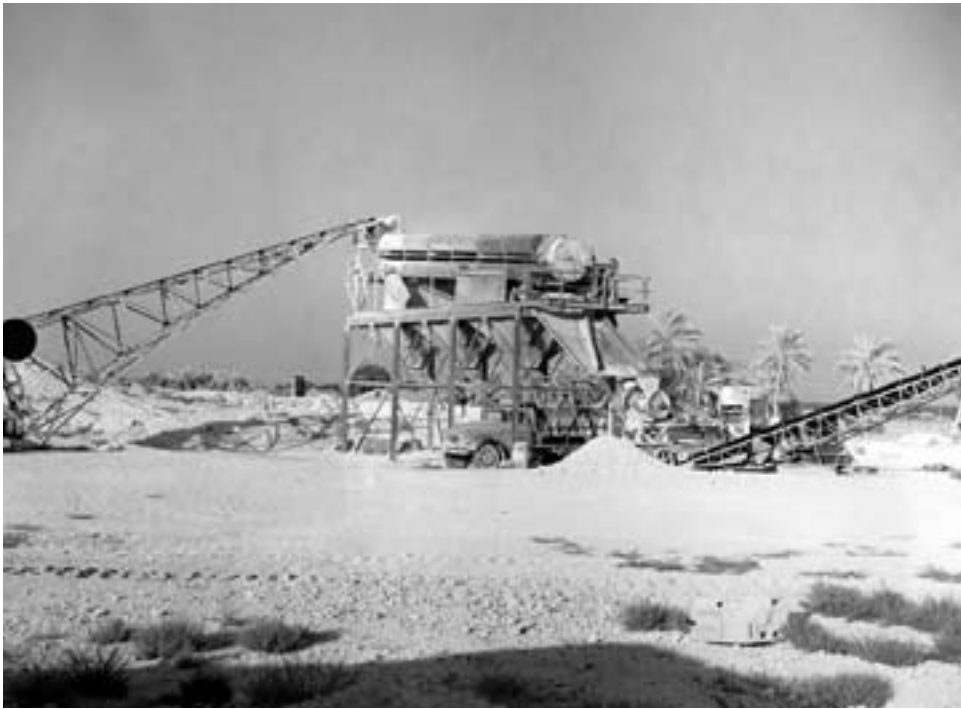
Rock-screening plant at Kharg Island
