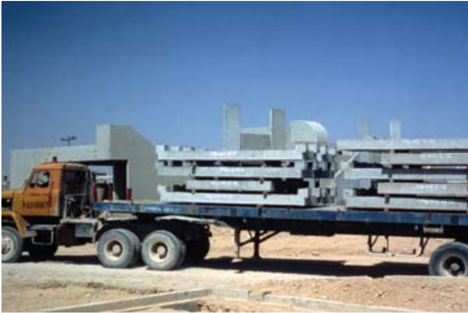
This page and top right, precast concrete panels were used extensively in construction at King Abdulaziz Military Academy.
