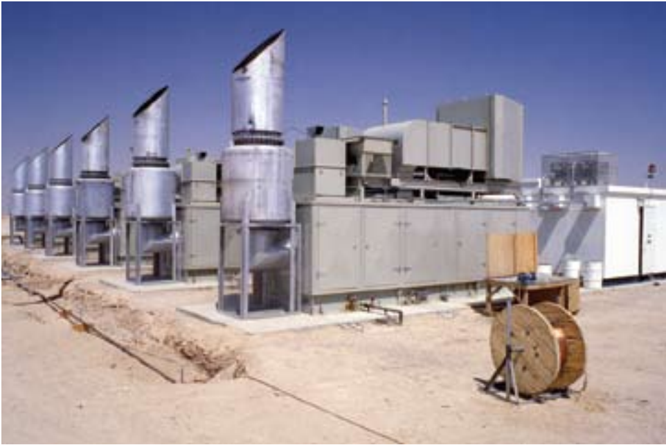
Generator turbines at Hafar al Batin
